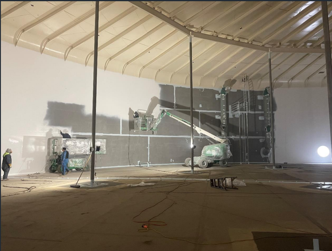
Coating by Spray Application
