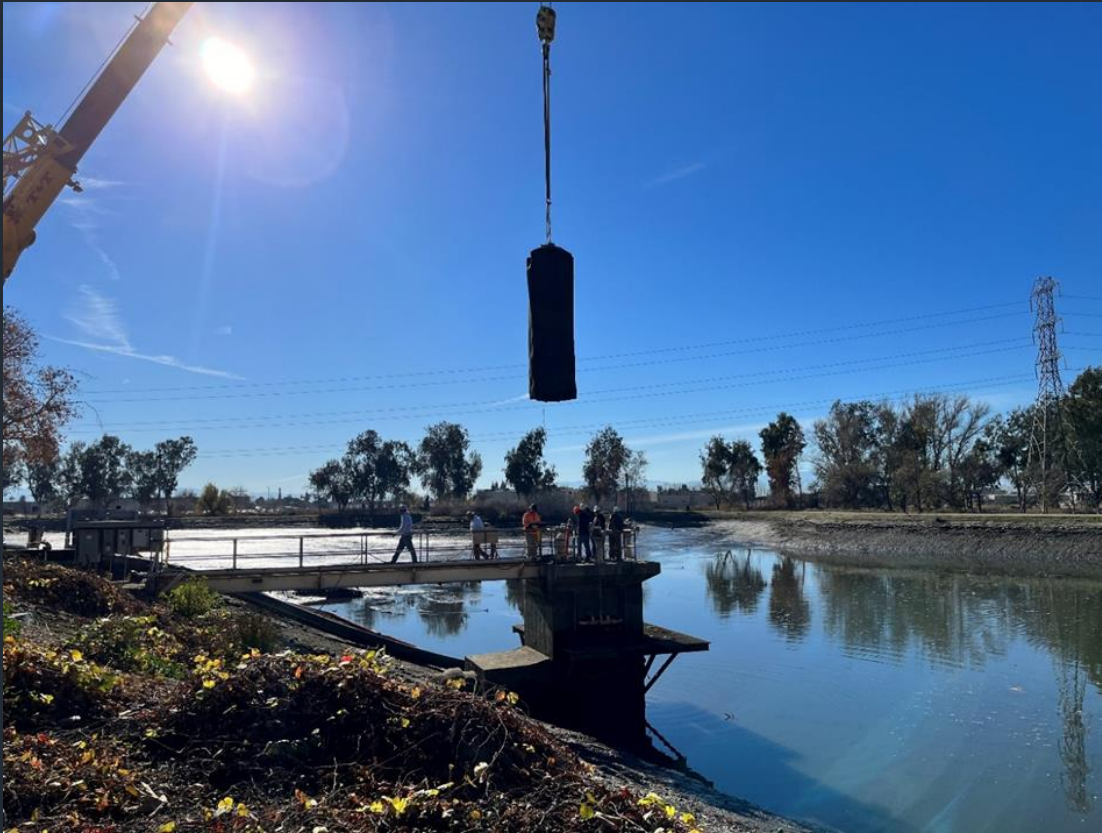
Lifting of 72" Pipeline Plug
