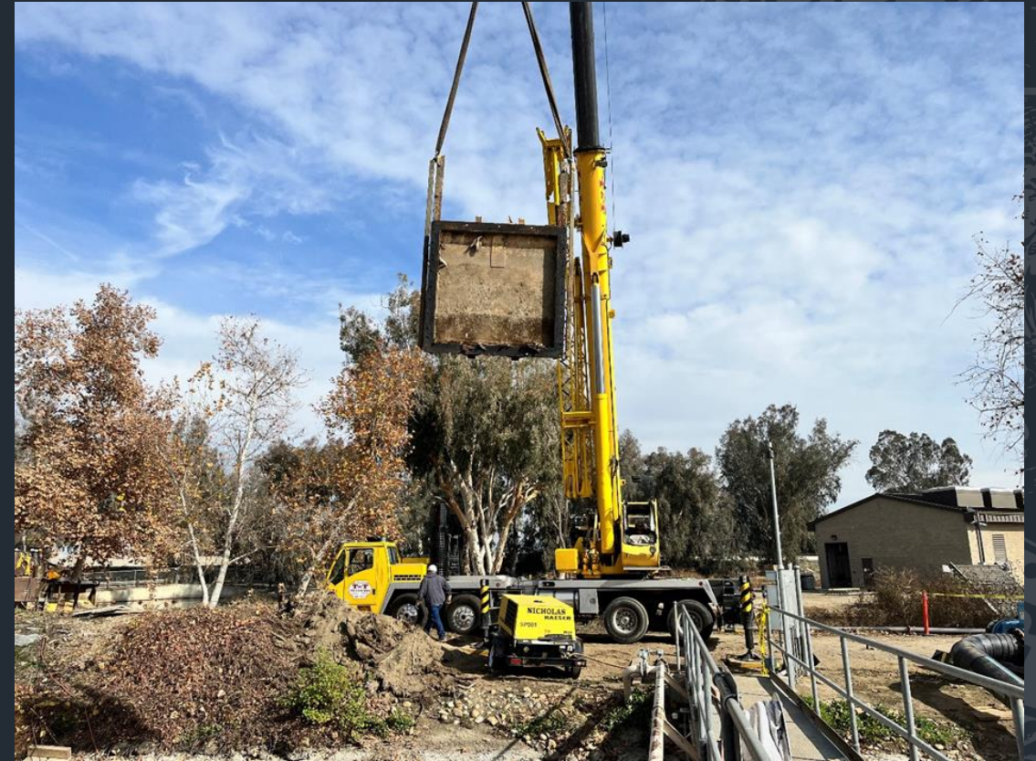
Removal of Existing Gate for Disposal
