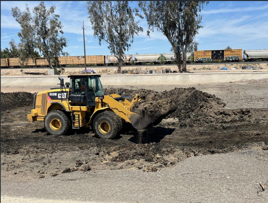
Removing Material from Drying Bed No. 9
