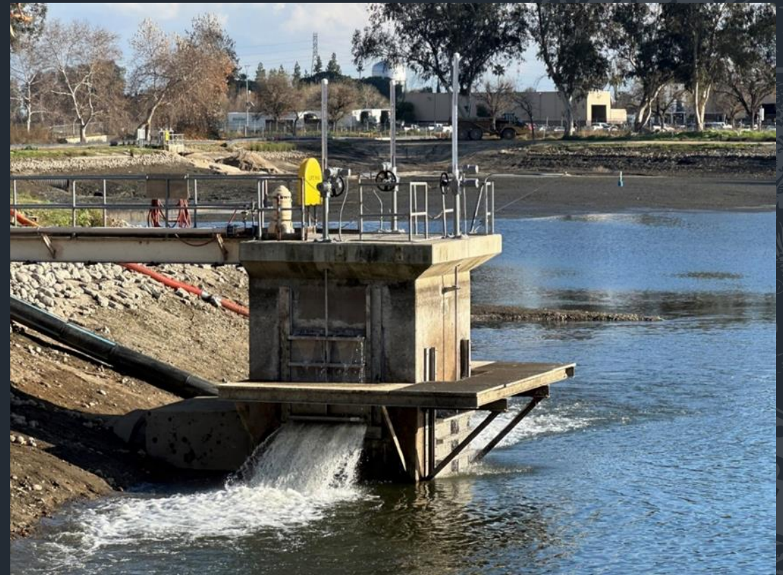
Removal of Plug
