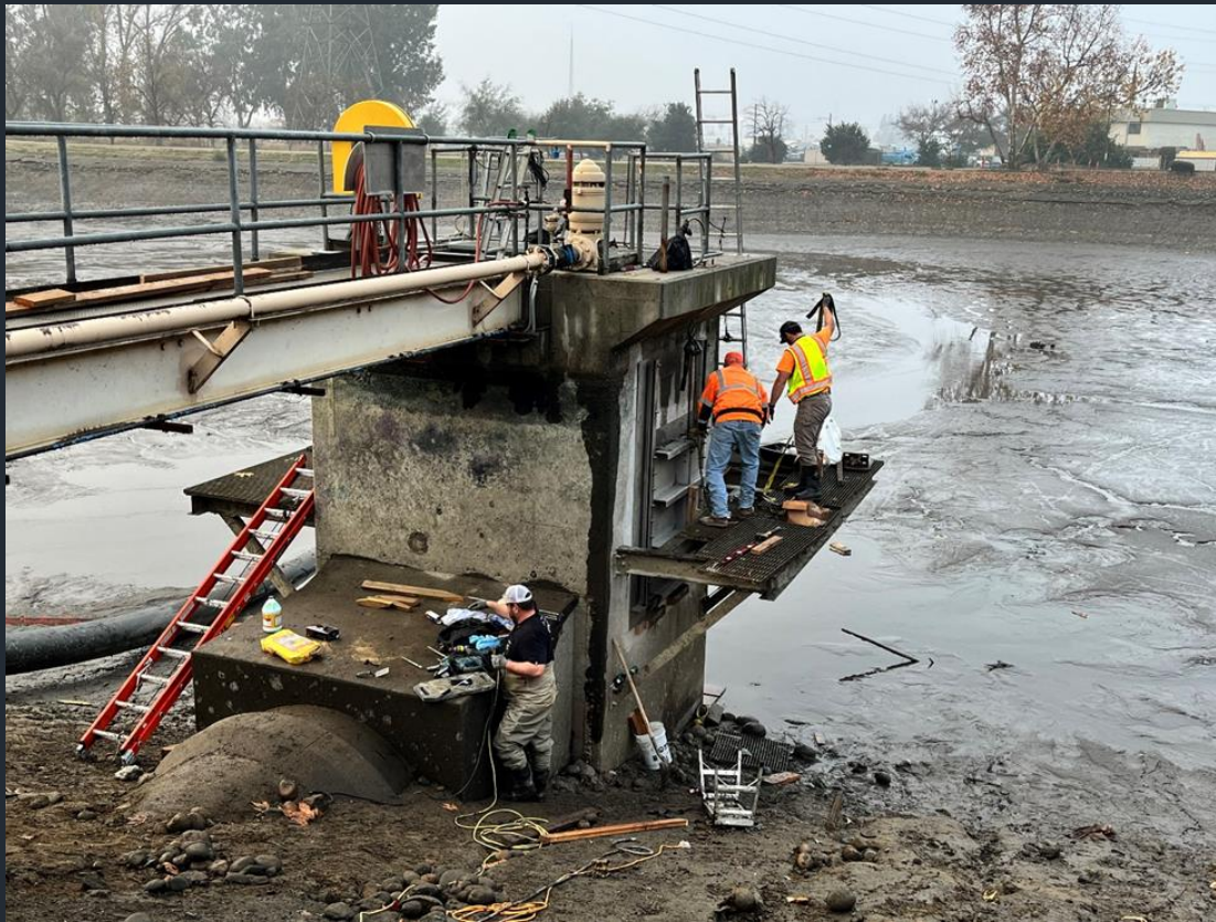
Installation of Gates
