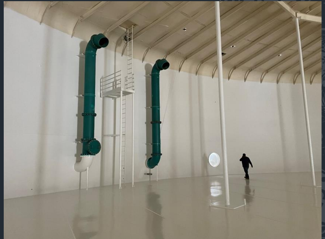
Completed Shell and Floor Coating (30-40 mils)
