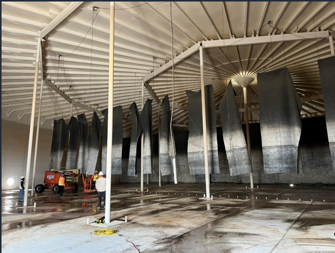
Removal and Disposal of Existing Baffle Curtains
