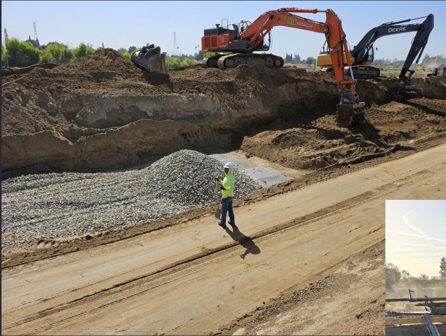
Compacting Fill & Placing Rock Foundation
