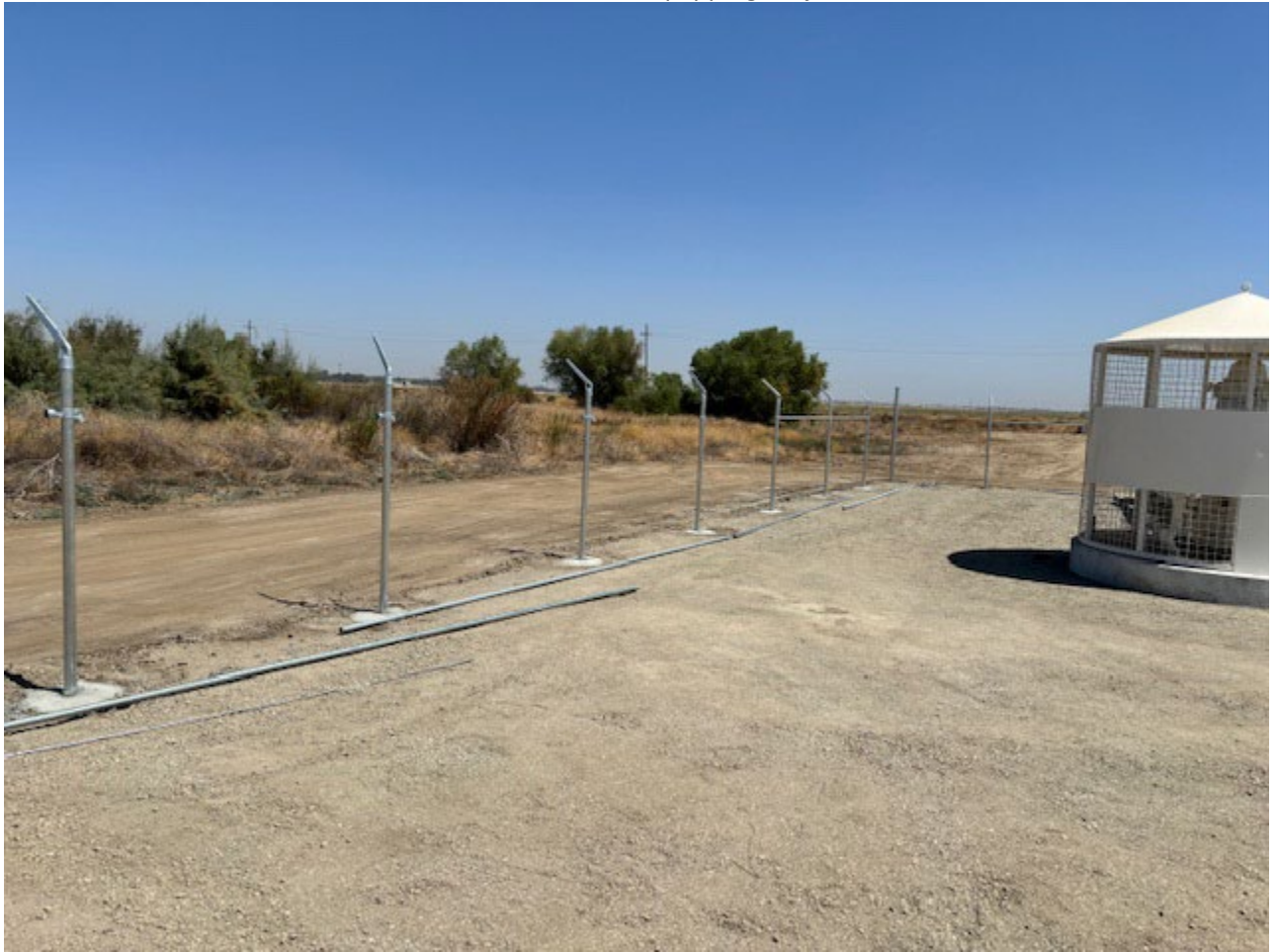
Installing Fence Framing at KCWA Well #39
