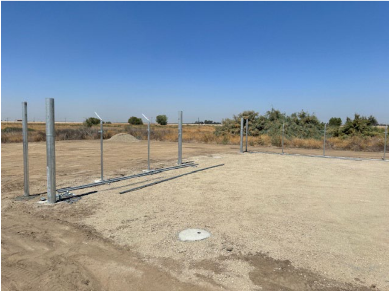
Installing Fence Framing at KCWA Well #39
