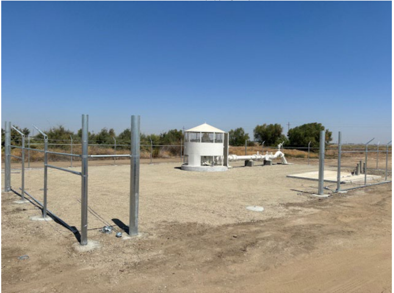
Installing Fence Framing at KCWA Well #39
